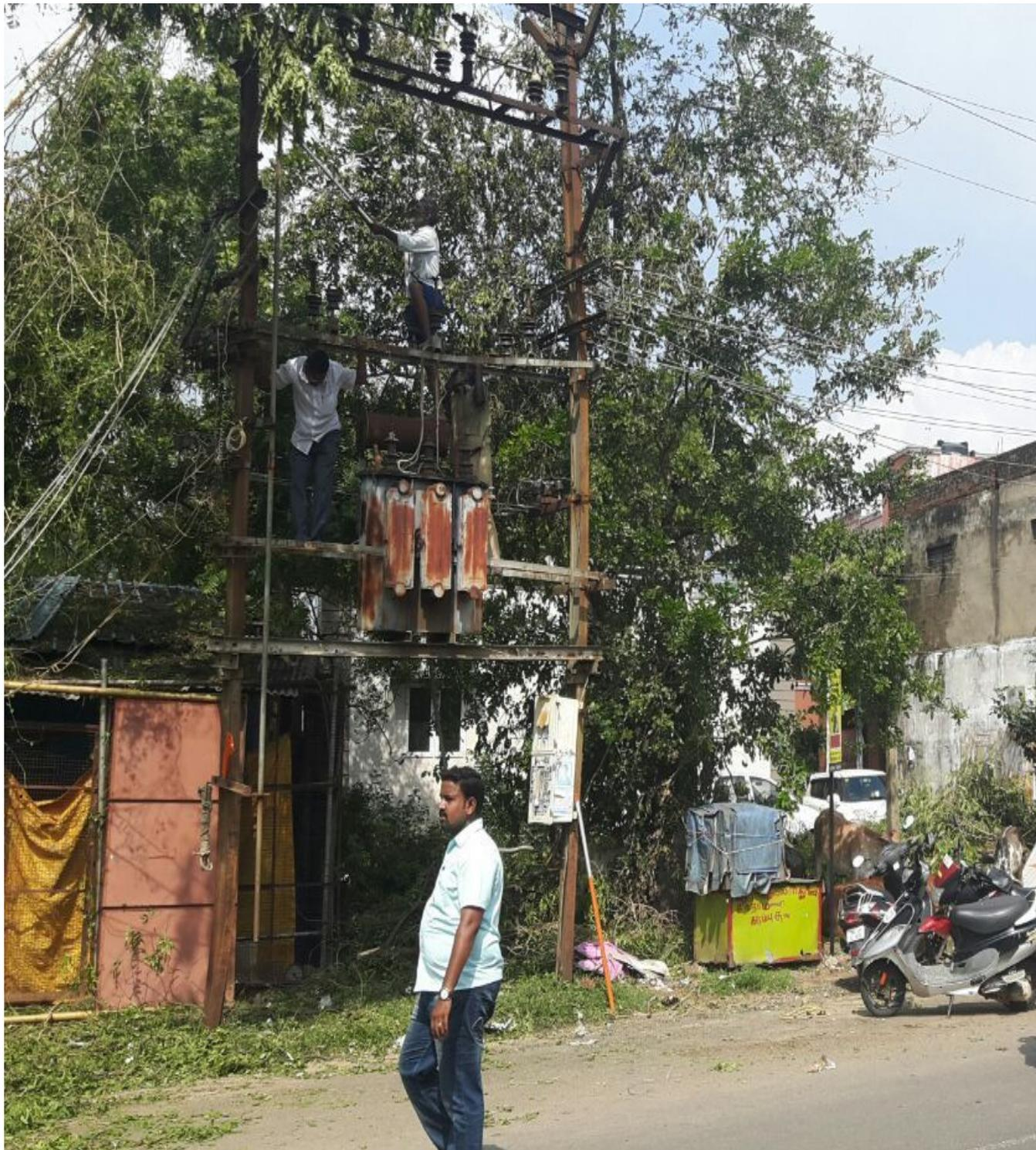
**Vardah Cyclone- Men at restoration work in Distribution Transformer Structure**
